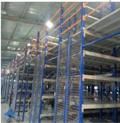
Steel Structure Support Mezzanine Floor
