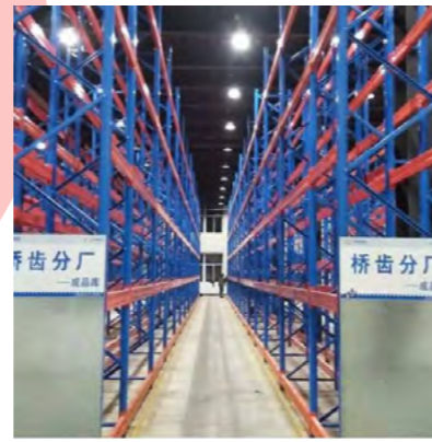
High Density VNA Storage Pallet Racking
