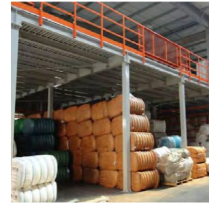
Multi- Level Platform Steel Structure
